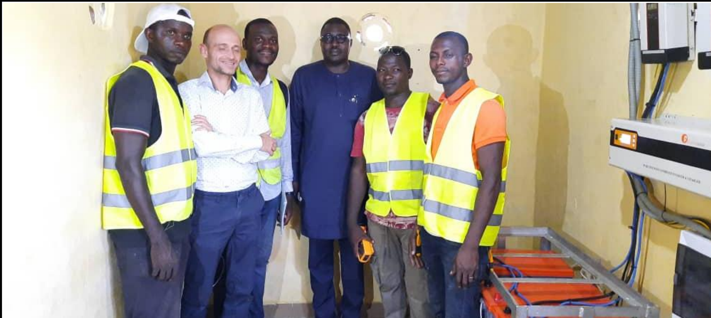
Power-Hub (Inverter & Battery Room)
